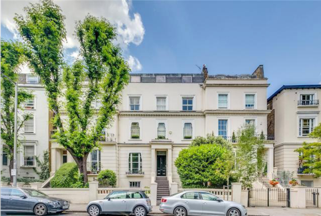
Image Courtesy of Blaze Fire Technology
